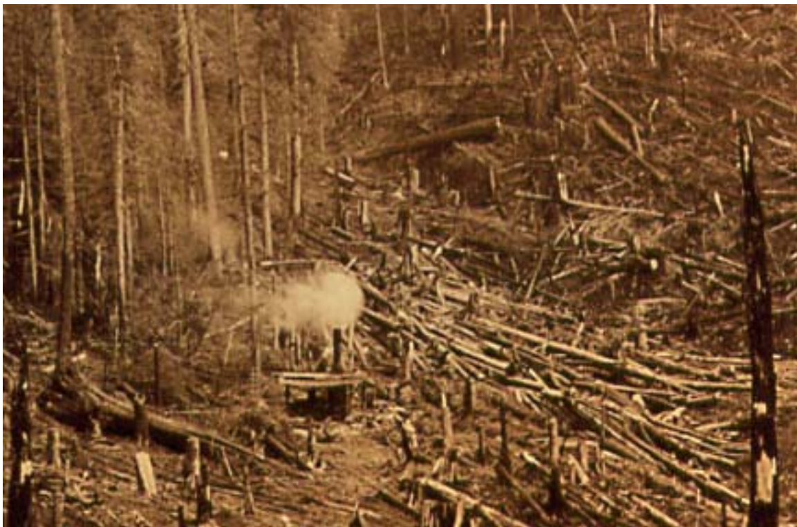
Clearing of forest for new Reservoir level.
