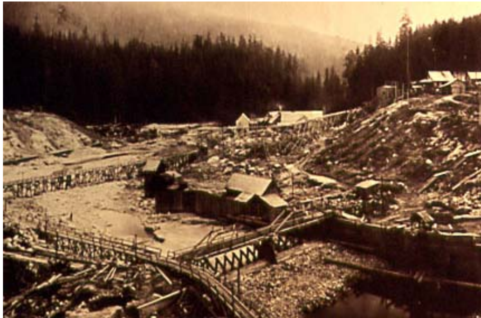
Beginning of construction period of second dam.
