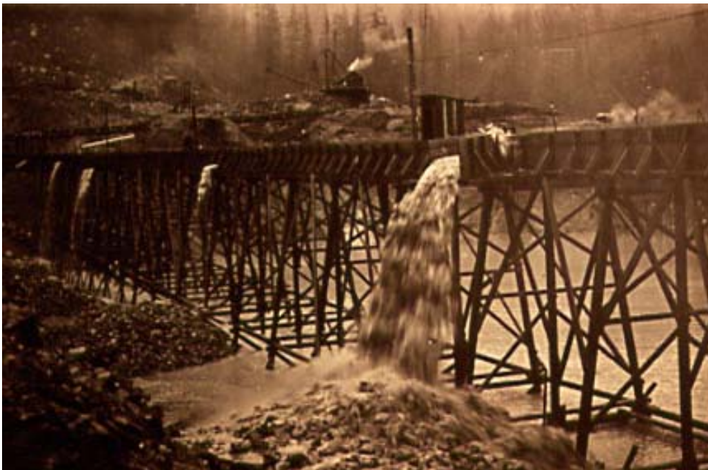
Sluicing platform and delivery of sluicing material for new dam. This period created many long periods of extreme turbidity in Coquitlam River, which residents often complained about.
