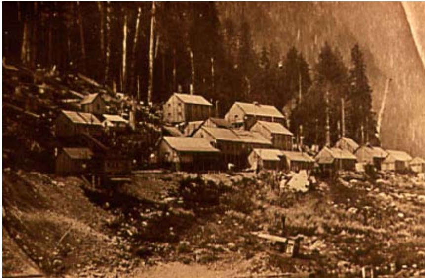
Tunnel construction residential and maintenance buildings.
