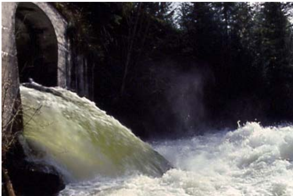
Diversion tunnel outlet at Buntzen Reservoir.
