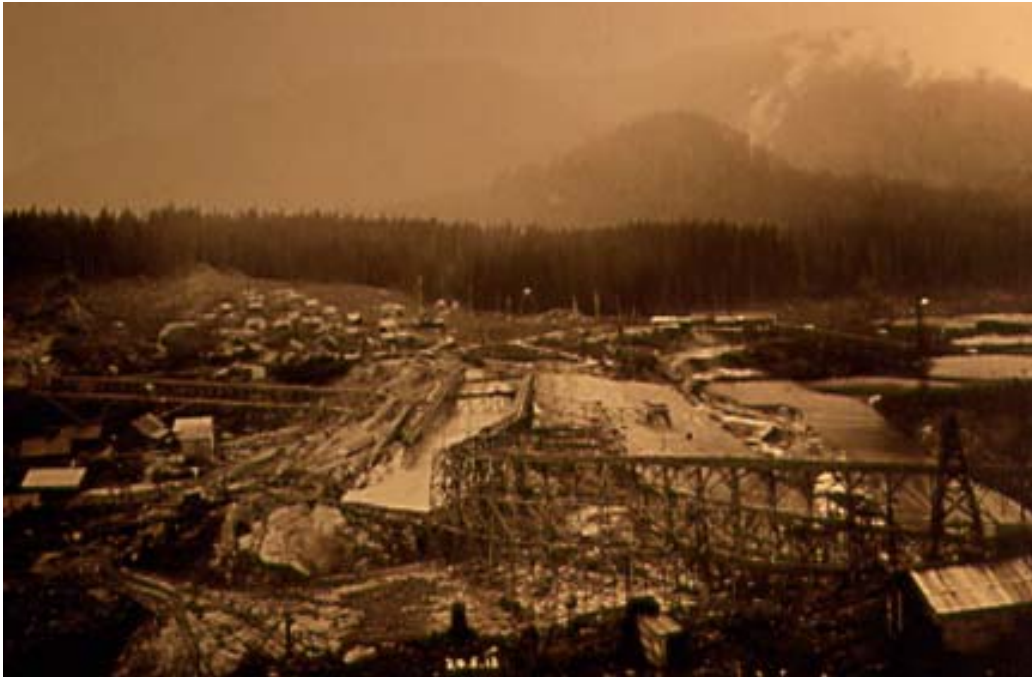
Final phase of Coquitlam dam construction. Photo taken May 20, 1913.
