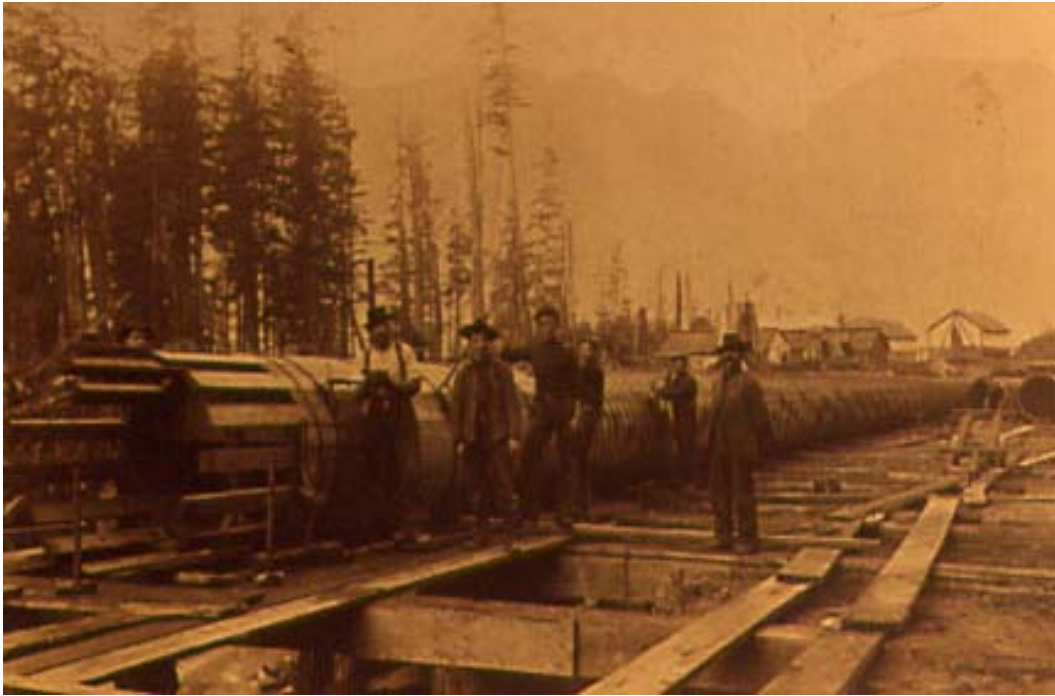
Wood-stave water pipe under construction from Coquitlam Lake.
