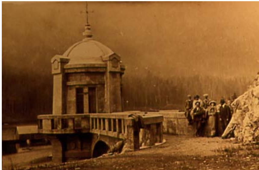
Newly constructed Coquitlam Reservoir water supply intake, around 1912. B.C. Hydro Archives photo.
