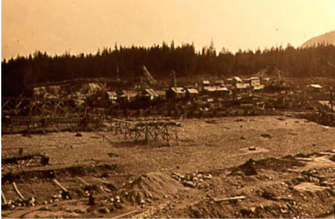
Housing complex during construction of second dam.
