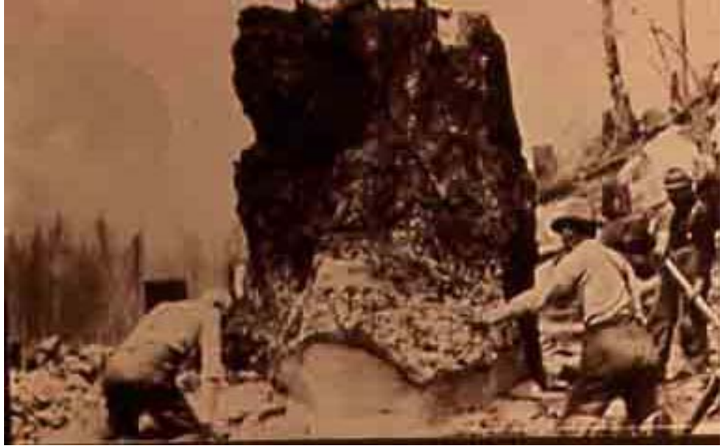
Photo of men cutting stumps down to one foot above ground level.
